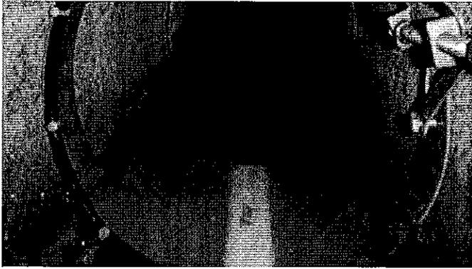
The CS4 Peak Combo sensor (at left) is our primary low-profile sensor for most standard manhole sites, and is installed in the invert of the pipe. This sensor includes three measurement technologies in a single housing: ADS' patented continuous wave peak velocity, up-looking ultrasonic depth, and pressure depth.
