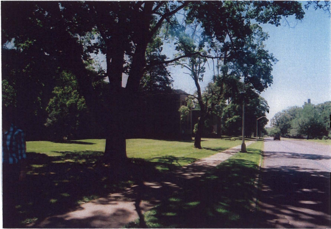
PHOTO 1: View south of the sidewalk, road and buildings 34 and 36 located within the northwestern portion of the project APE. The National Register Eligibility site form indicates the structures were constructed in 1930 and served as patient housing and for patient services.
