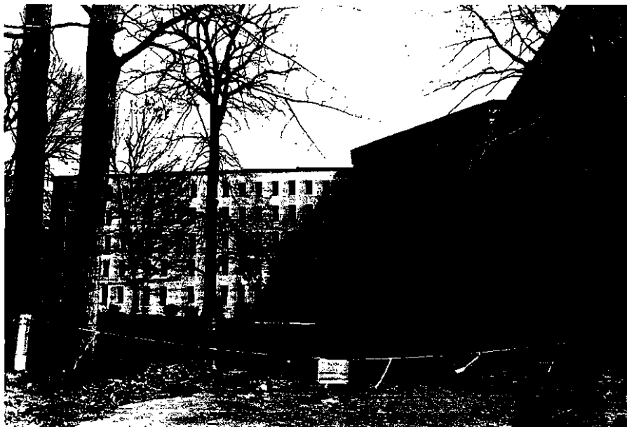
Bldg.60 looking east
