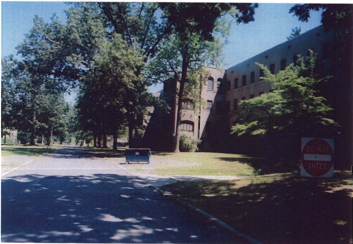
PHOTO 2: View north of the road and buildings 4, 7, and 8 located within the west central portion of the Psychiatric Center complex. The buildings were built in 1927 and used for medical services and as dining rooms and clinics.
