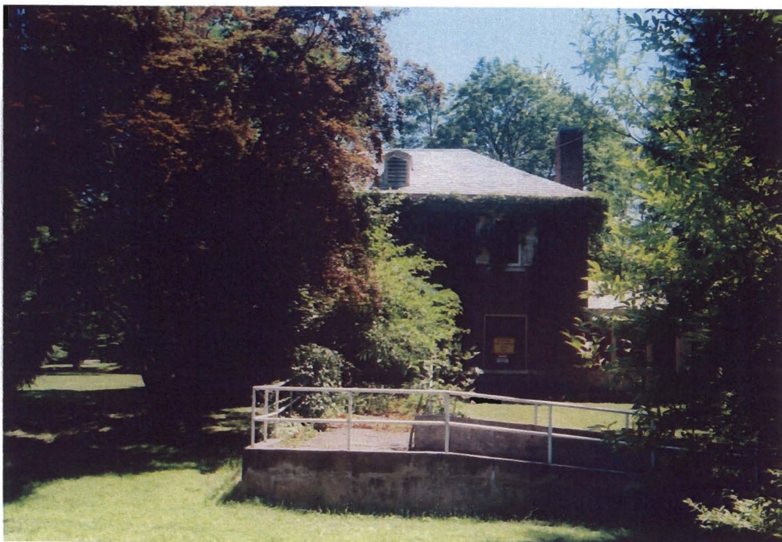
PHOTO 12: View southwest of building 52 located along the south side of Old Orangeburg Road within the southern portion of the APE. The structure is not listed in the building-structure inventory.
