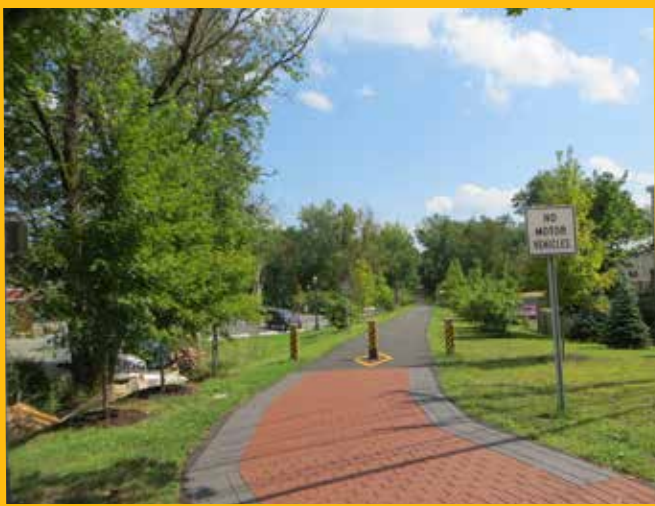
ROAD TRAIL INTERSECTION IN SPARKILL
