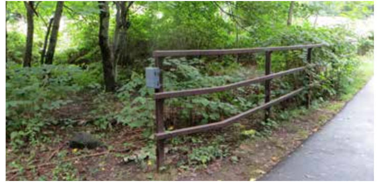
PYRO BOX COUNTER INSTALLED AT SPARKILL DEPOT
