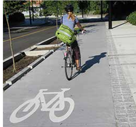
A NEWLY-CONSTRUCTED SIDEPATH
