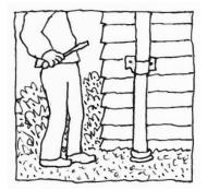
First, secure the downspout to the wall with a clamp screwed or nailed snugly to the siding.
