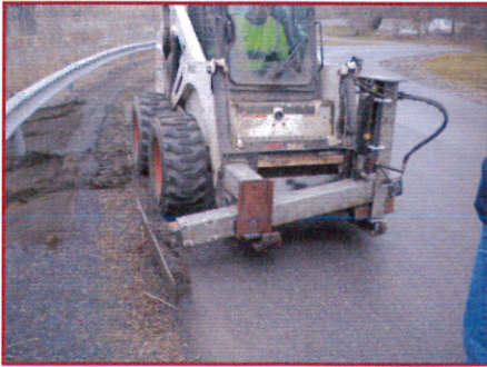
Town of Ulster Under the Guidrail Cleaner
