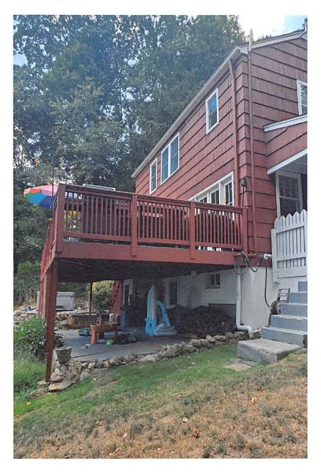
**4. Existing Deck as Viewed From The North.** The unusable higher slab under the deck is evident. Stairs from the north porch to grade will be removed. The porch setback from the east house elevation will remain.
