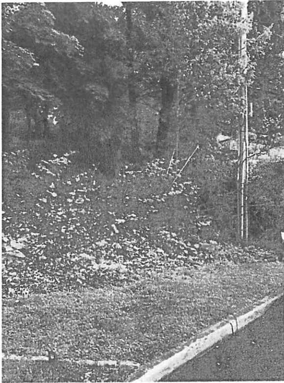
Utility pole with underground feeds and property line approx. location
