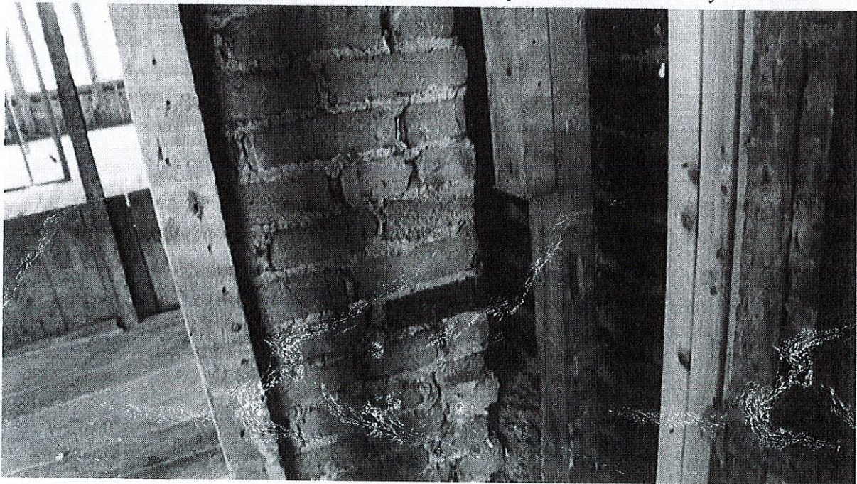
This is an abandoned brick chimney that is structurally unstable and does not have proper support in the basement. We propose removing this. It is not a significant architectural element from the street and is barely visible mainly due to the large pine tree in front.
