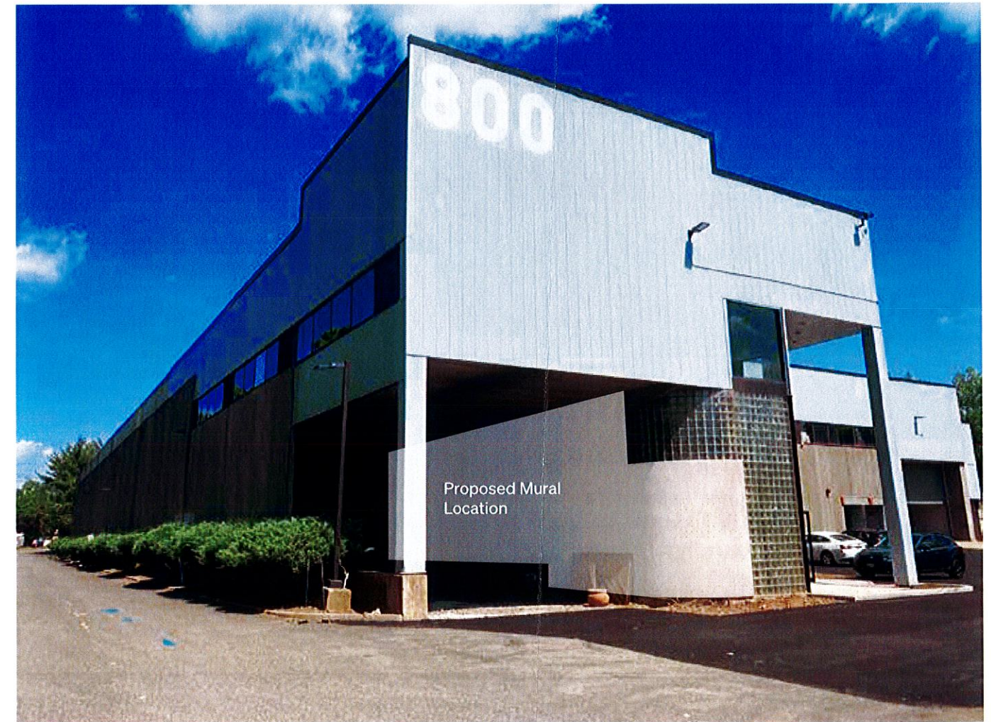
Photo of existing conditions
