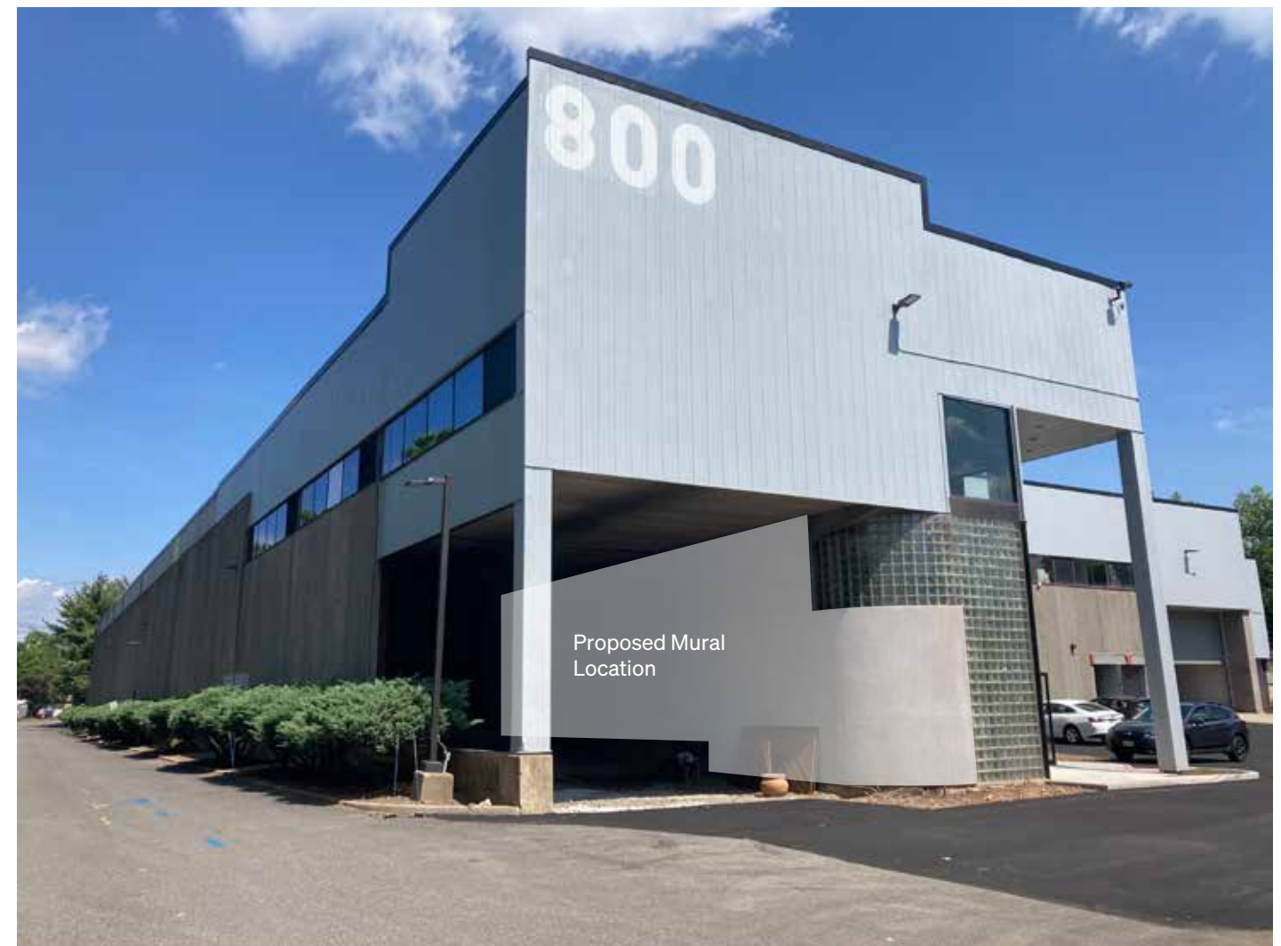
Photo of existing conditions
