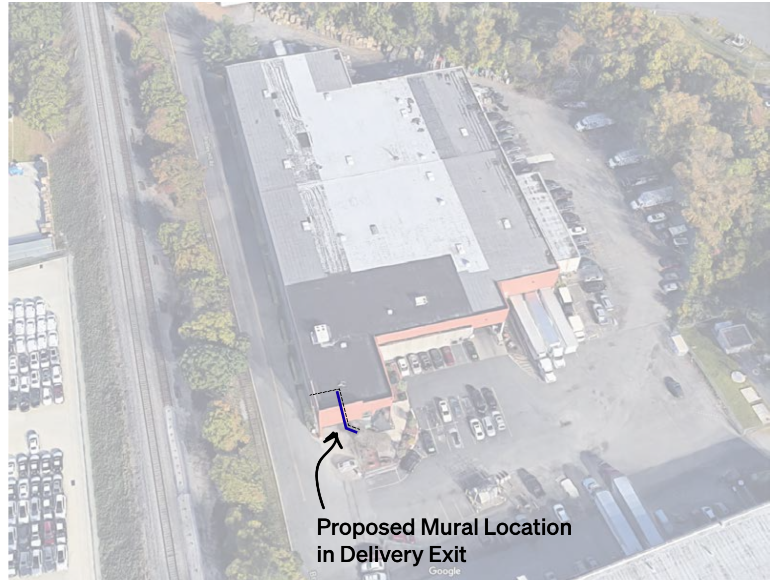
Satellite View of Building
