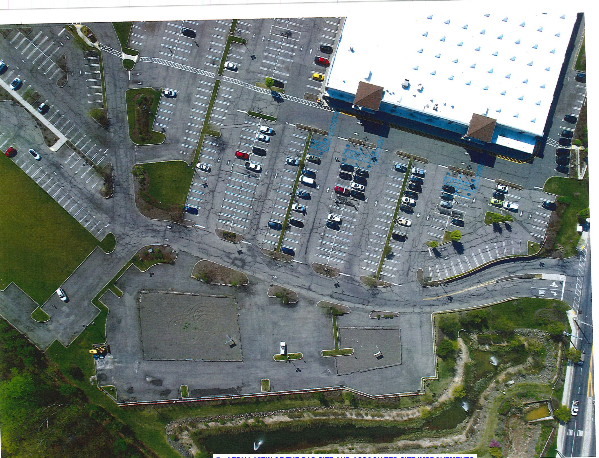
7 - AERIAL VIEW OF THE PAD SITE AND ASSOCIATED SITE IMPROVEMENTS
