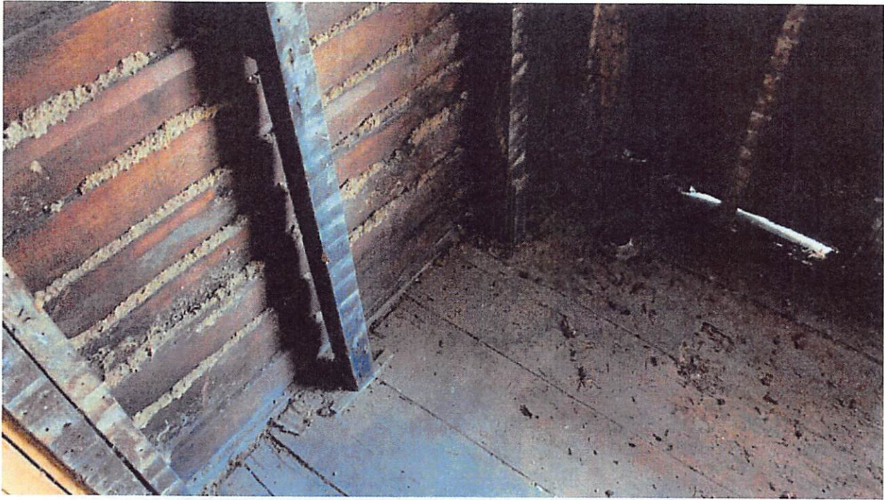
Here is a closer look at the west wall construction from inside. Note the daylight coming from under the north wall. Although not visible here due to old cellulose insulation blocking it, there is daylight coming in between the exterior clapboards as well in many locations.
