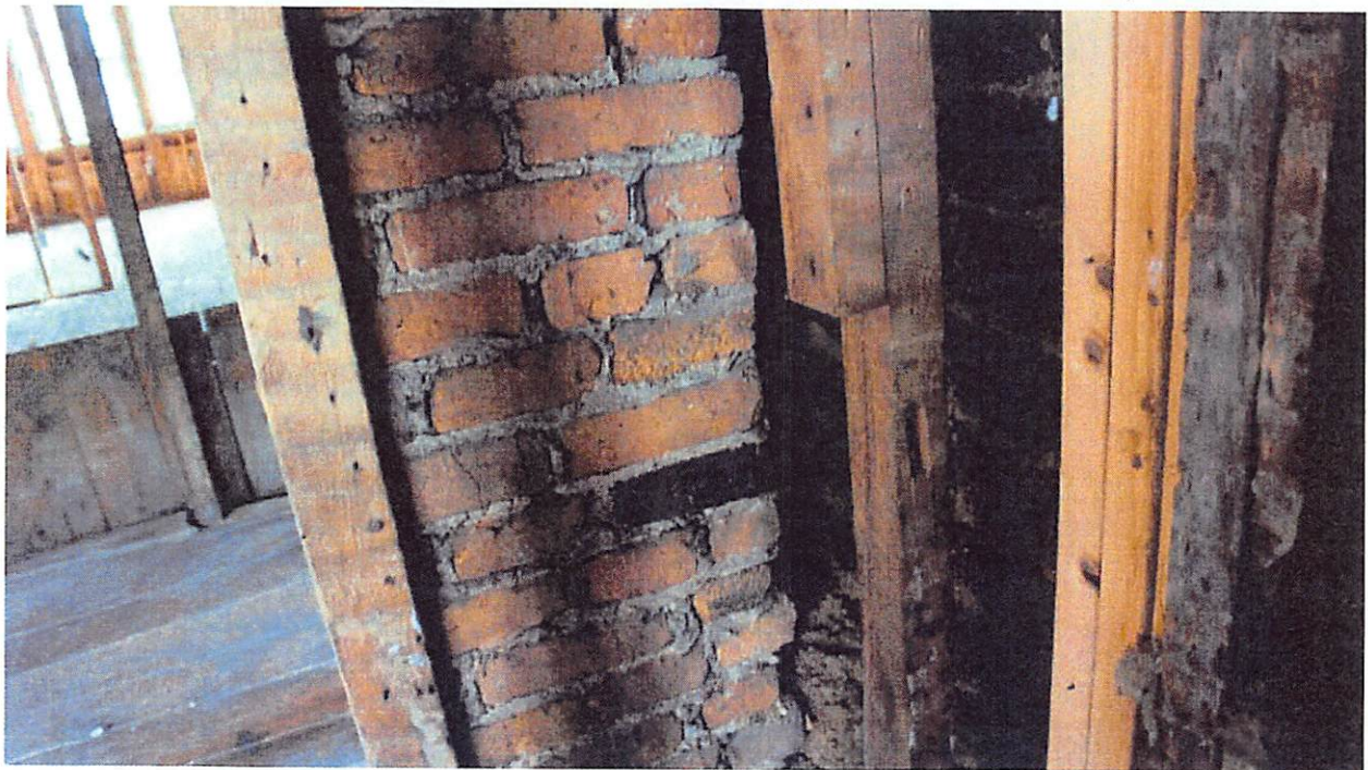
Here is a closer look at the west wall construction from inside. Note the daylight coming from under the north wall. Although not visible here due to old cellulose insulation blocking it, there is daylight coming in between the exterior clapboards as well in many locations.
