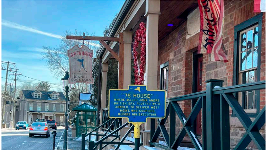
110 Main Street, Tappan ("76 House") © AKRF
