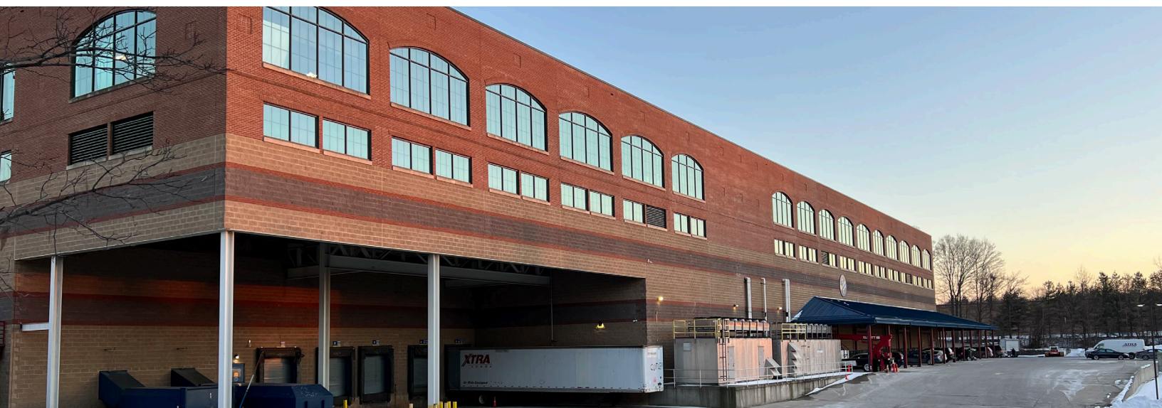
Industrial Park, NYS Route 303 © AKRF
