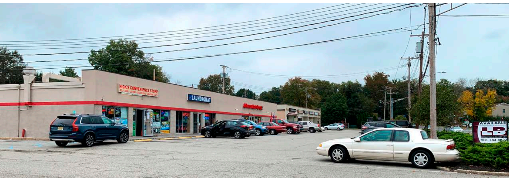
Commercial storefronts on Route 303, Tappan © AKRF
