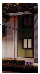
In the areas where there is one window on top of the other, the siding will be replaced with this green board and batten vertical siding.
