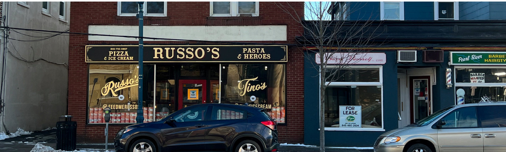
Commercial corridor in downtown Pearl River © AKRF
