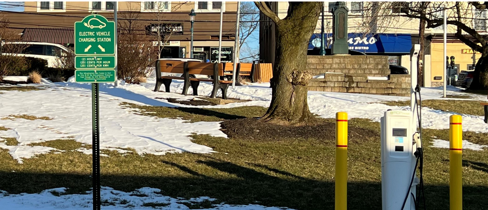
Electric vehicle charging station, Pearl River © AKRF
