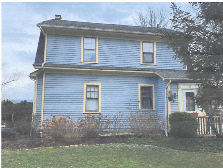
West elevation – addition location
