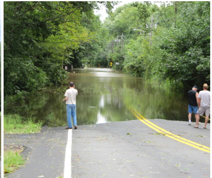
Oak Tree Road after Hurricane Irene 35
