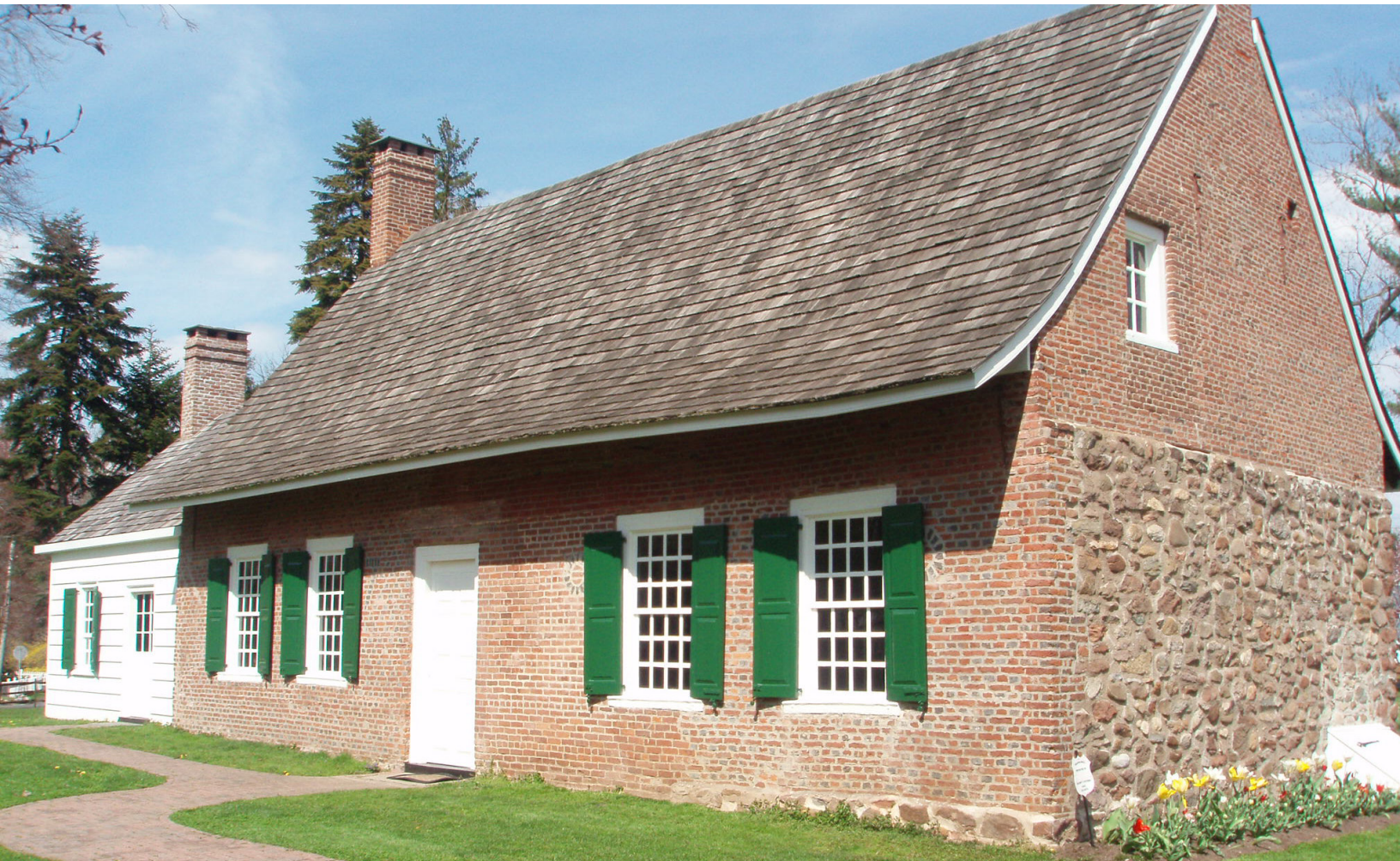
Dewint House, Tappan, built 1700. Source: WikiCommons
