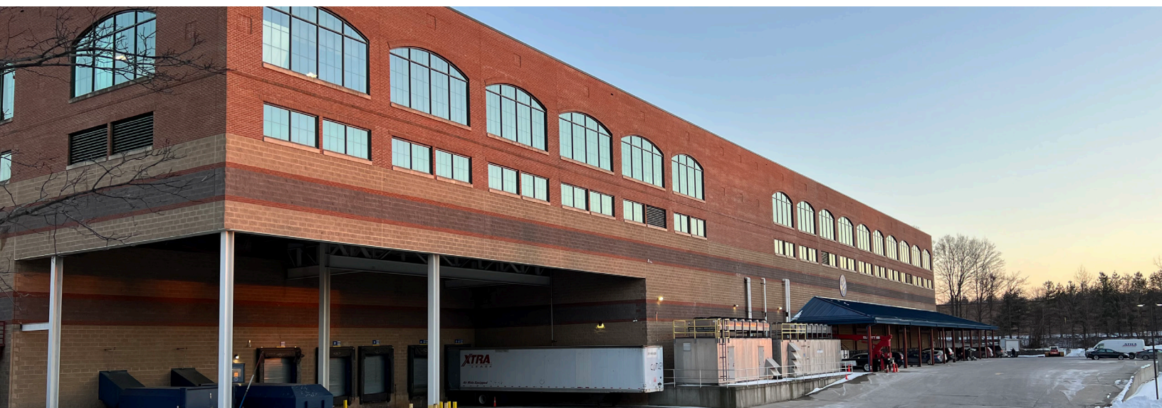
Industrial Park, NYS Route 303 © AKRF
