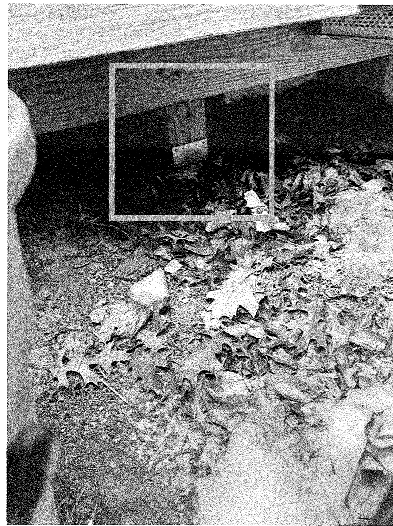
PHOTO 1 - POSTS ON CONCRETE FOOTING
