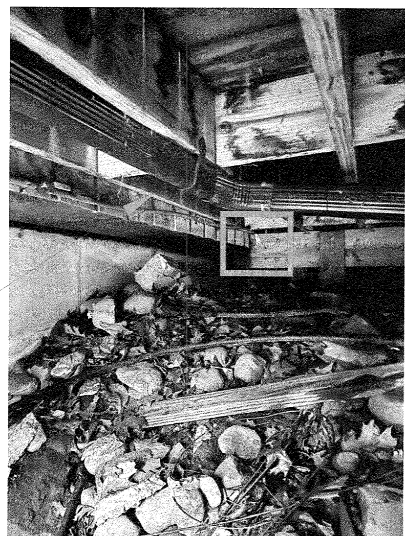
PHOTO 4 - LEDGER AT PRIMARY STRUCTURE & TIE BACK
