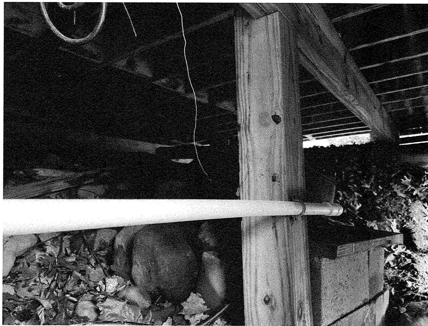
PHOTO 3 - TALLEST POST, BEARING, BLOCKING
