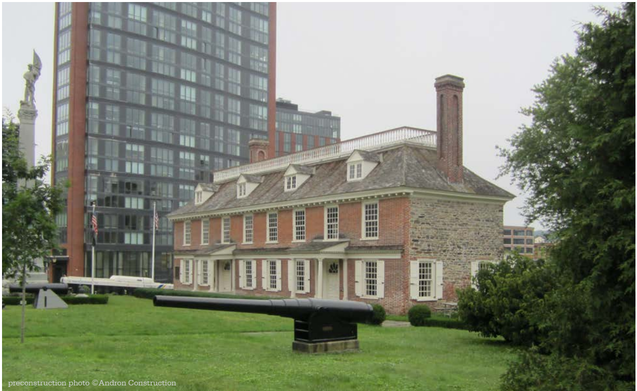
preconstruction photo ©Andron Construction
