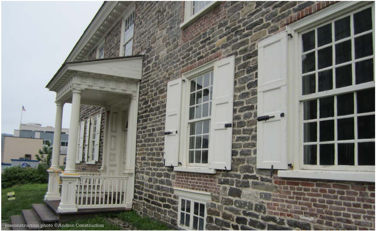
preconstruction photo ©Andron Construction
