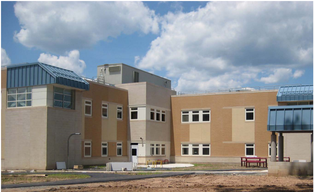
construction photos ©Andron Construction
