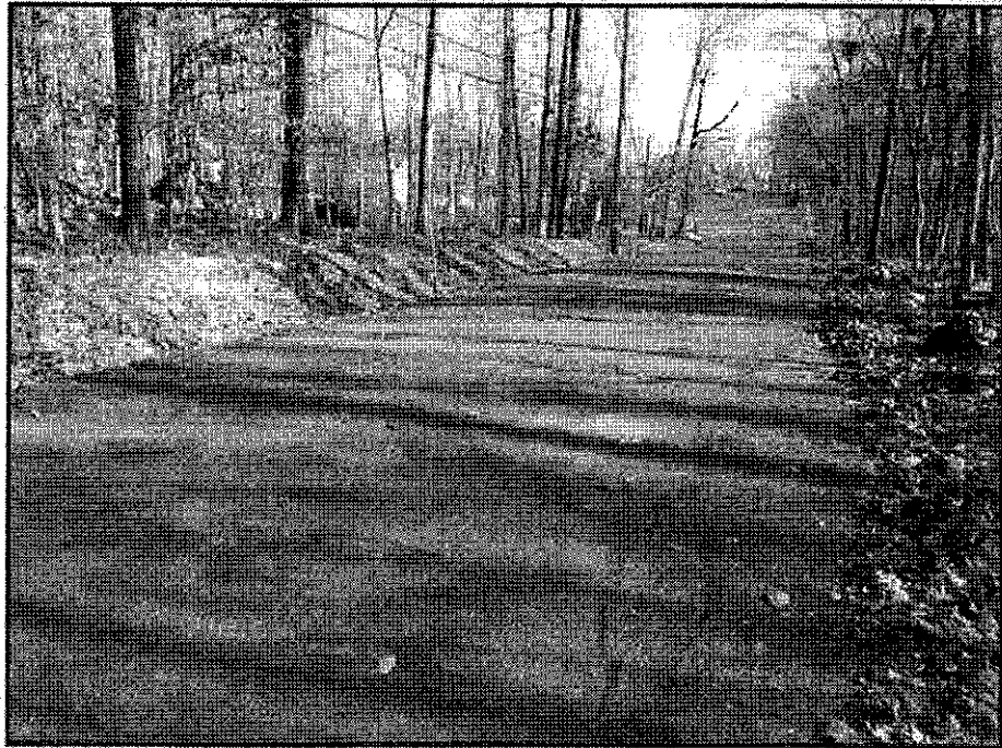
Gatto Lane at Site Access Drive, Looking East
