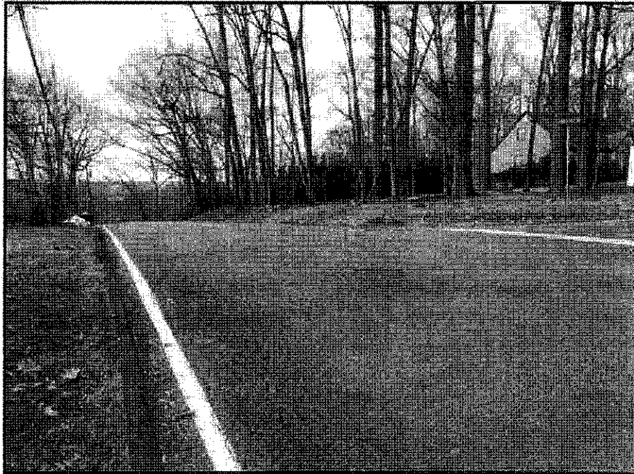
Crooked Hill Road at North Highland Avenue, Looking West
