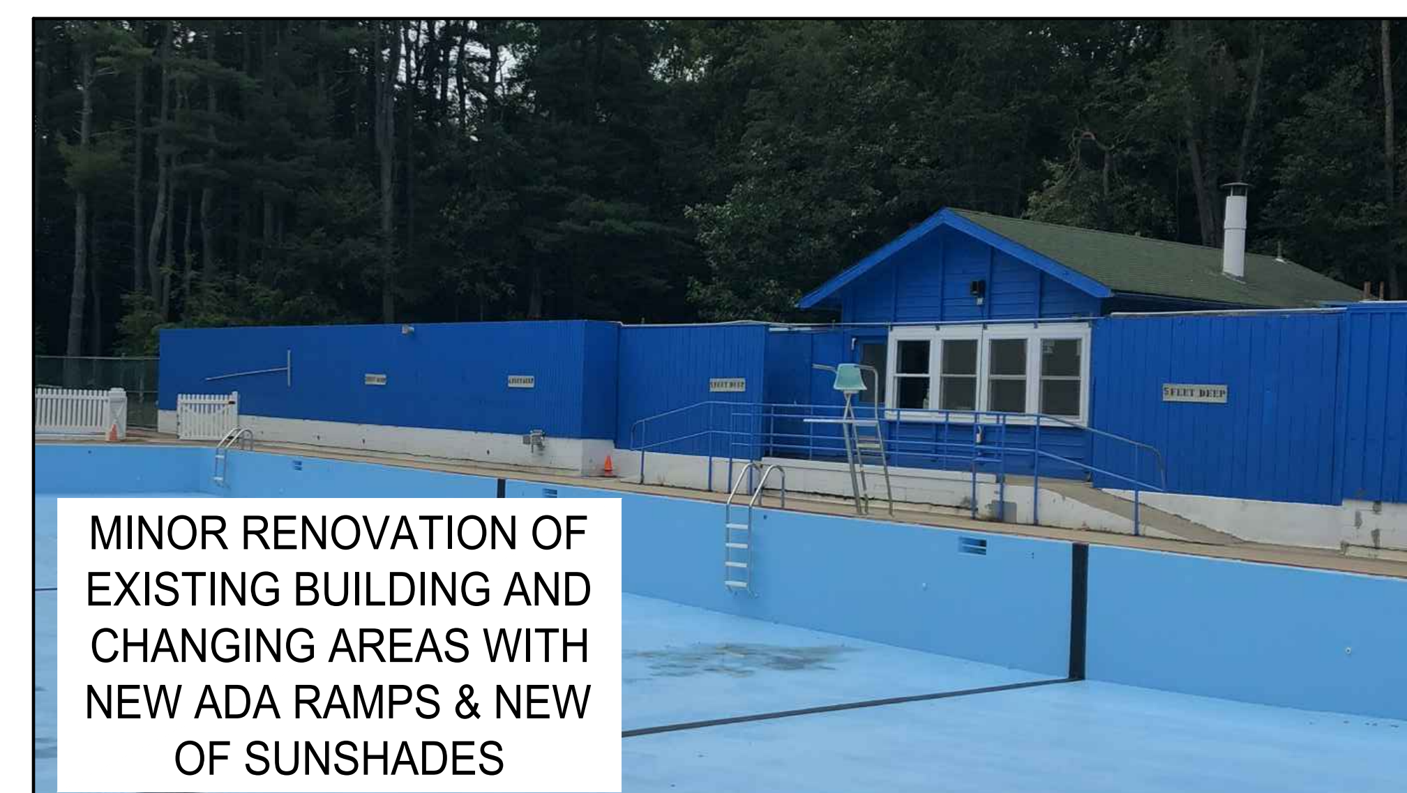
1 EXISTING AQUATIC CENTER & LIFE GUARD STATION
