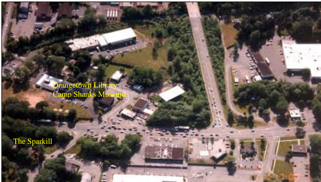
This aerial overview of the Orangeburg Road intersection with Route 303 illustrates several open space opportunities, including the Sparkill streambed and the Camp Shanks Museum and Orangetown library.
